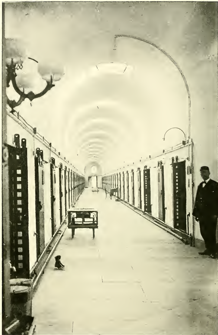
Ninth Block—254 ft. long, 10 ft. wide, 16 ft. high—50 Rooms, 18x8 ft., 12 ft. high— Eastern State Penitentiary.
